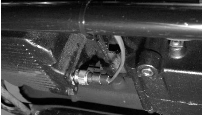
Installed oil temp sensor and harness plug
